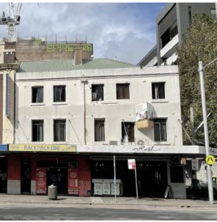
Subject Site 238-240 Reservoir Street
