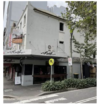
Subject Site 238-240 Reservoir Street
