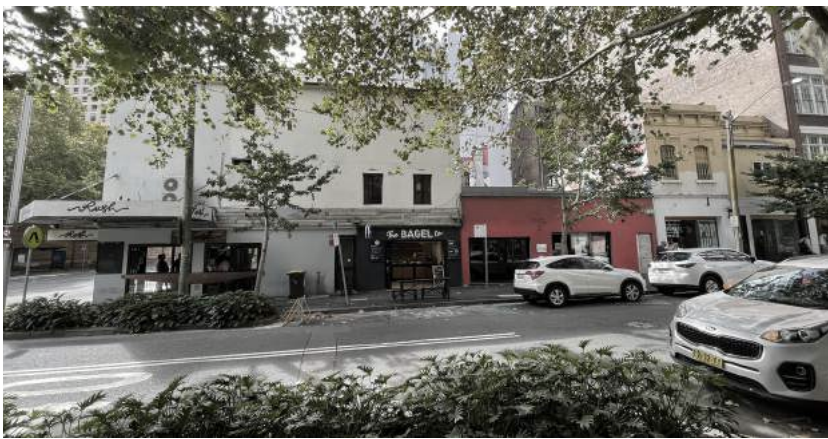
Subject Site 238-240 Reservoir Street
